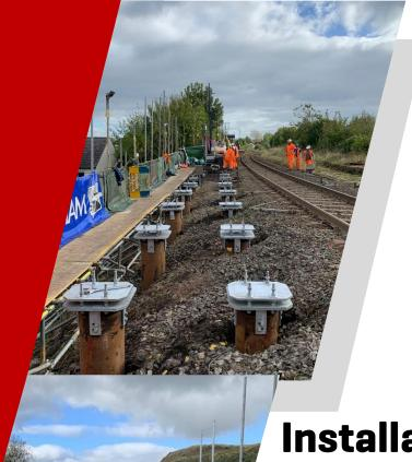
Installation of CHS piles for new station platform
